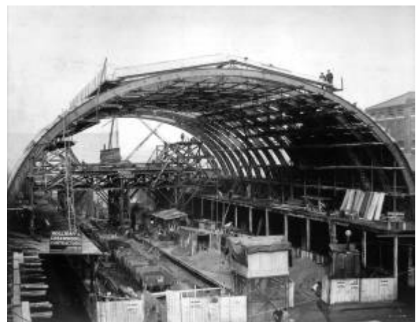
Span Four under construction (Staffordshire Record Office)
